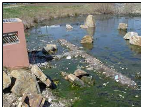
Low Flow Device uses a T-Connection and Runs Parallel to the Side Slopes
