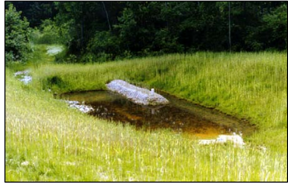
The low flow device is visible above the water surface and is unattractive
