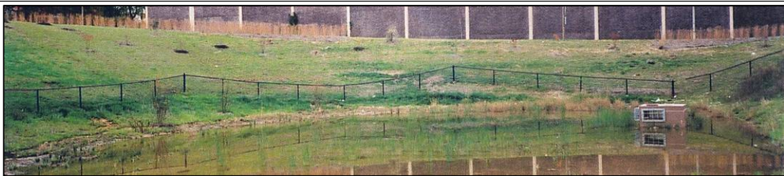
Fence Steps Up and Down Contours (Avoid)
