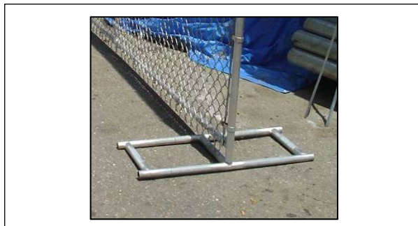
Figure 5-4. Footer at Temporary Fencing
