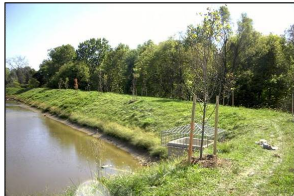
Example of stormwater facility with trees planted along the embankment. This can cause damage to the embankment and ultimately cause embankment failure.
