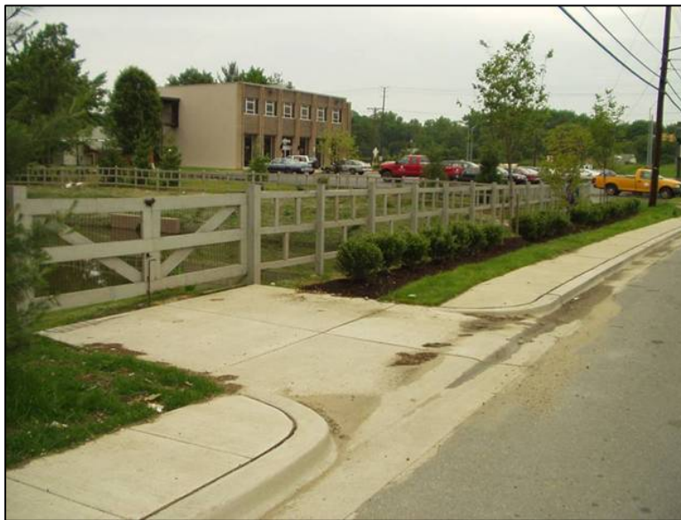
Figure 6-7. Concrete Apron and Depressed Curb Provided at Maintenance Access
