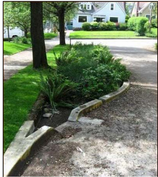
This curb extension filtration strip helps to improve water quality and aesthetics while also providing traffic calming. Photo Credit: EPA
