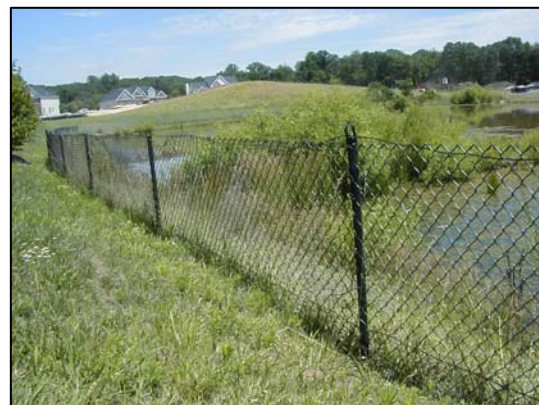
Black Vinyl Coated with Tension Wire
