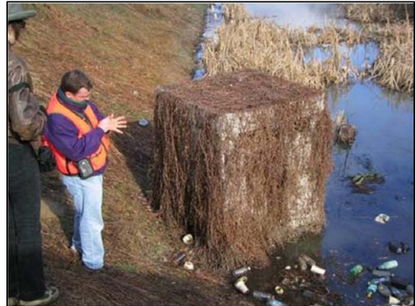
Woody vegetation, including ivy, must be kept clear from a riser structure to ensure proper function.
