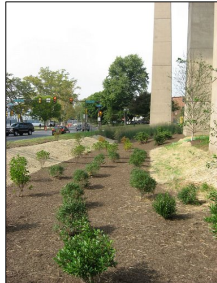
Example of a facility with Type A Matting used on side slopes. Photo Credit: EPA
