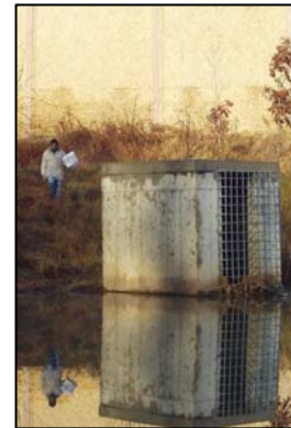
This riser does not meet safety criteria because of its excessive height.
